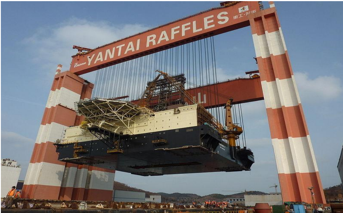
The most powerful crane Taisun
